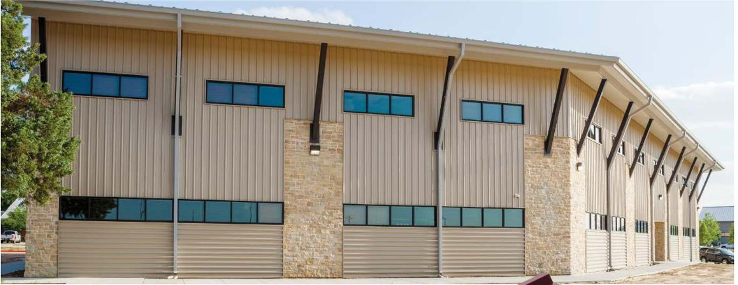
The Berridge "R" Panel is a wide, economical panel providing 36" of coverage for vertical or horizontal applications. Similar to the "M" Panel, this exposed fastener panel provides a different pattern option for a wide range of applications.
