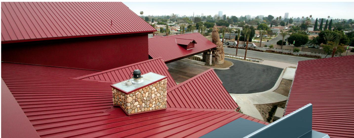
The Berridge Double-Lock Zee-Lock is a 2" high standing seam panel with 16" coverage and is 180-degree mechanically seamed. This panel can be installed over open framing or solid sheathing and is available in both steel and aluminum making it ideal for multiple applications.
